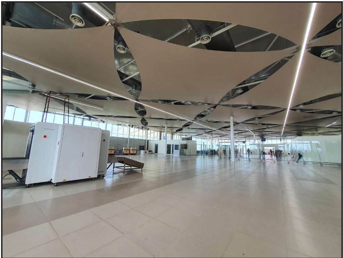
X-BIS Machine Installed at Kushinagar Airport
